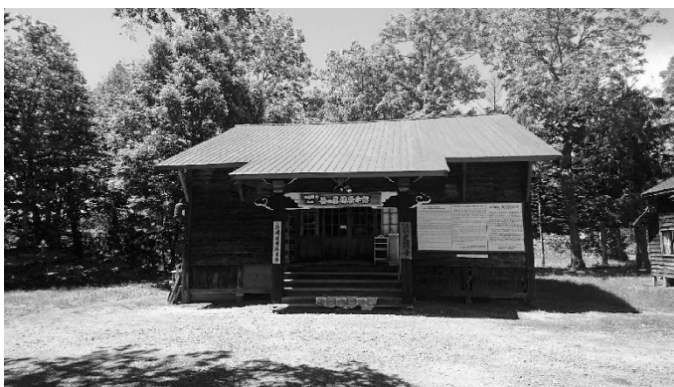
Figure 1: Former Sasa No Bohyo Exhibition Hall 3)
