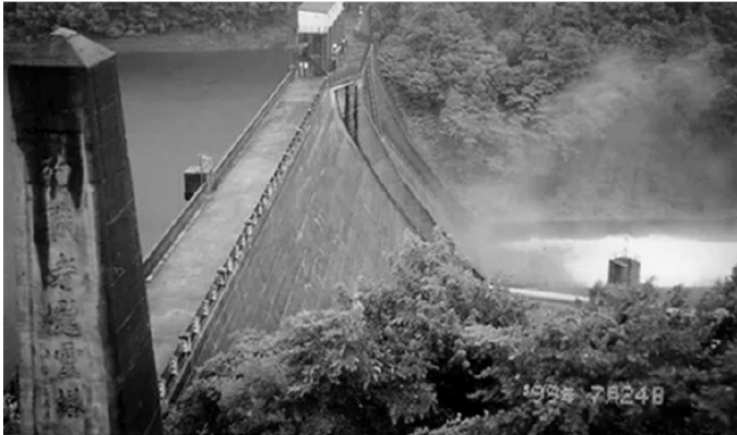
Figure 2: Uryu Dam in Shumarinai
